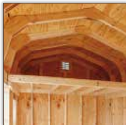
4' Deep Loft in Dutch Barn
