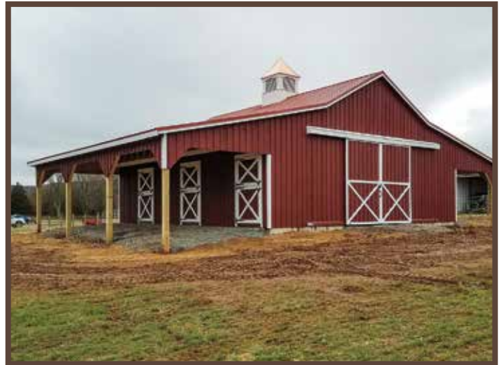
(523) On-Site Build Horse Barn
