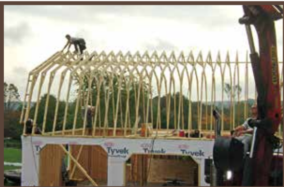
Build On Site
